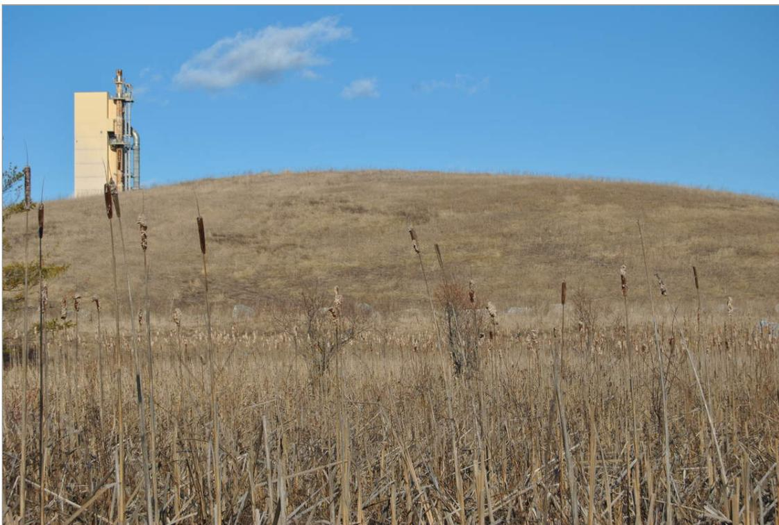
The waste kiln dust pile, partially covered in clay, soil and grass, fills an old quarry at the southeast corner of Dragon's property and is bordered by a wetland.
